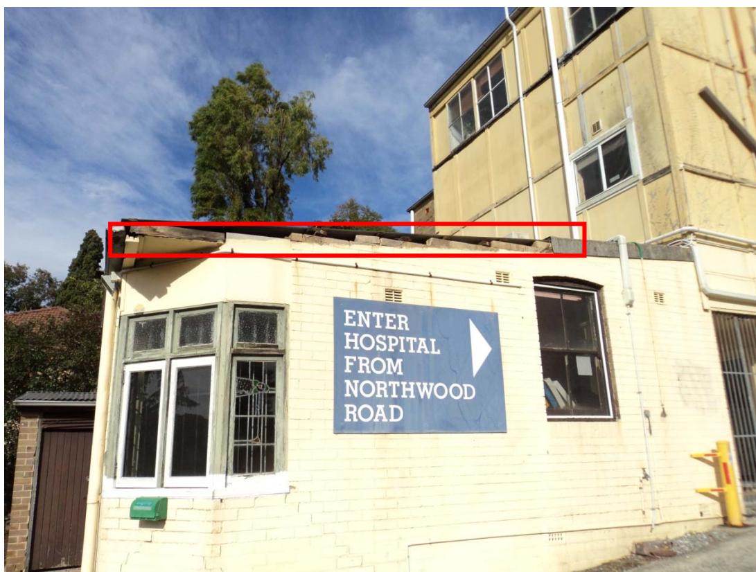
Photograph 10 Crevices in roofing (outlined in red) suitable for microbats
